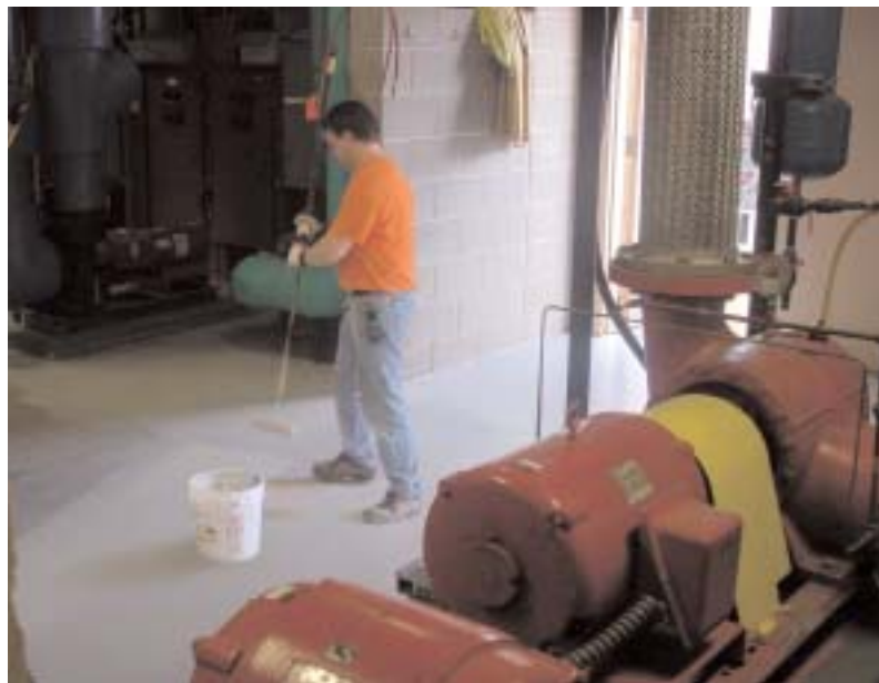
MCI®-2026 Flooring System combines the strength of our concrete primer and floor coating.
