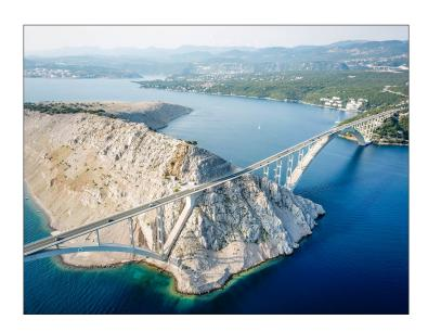
The Krk Bridge, which includes one of the world's longest reinforced concrete arches, is located in a corrosive environment where strong winds blow salt spray onto the bridge's surface. Almost four decades of chloride exposure led to corrosion problems that, due to inadequate maintenance, threatened to endanger the bridge's stability unless proper preservation measures were taken. With one million vehicles traveling across the bridge every year, mitigation was critical.
