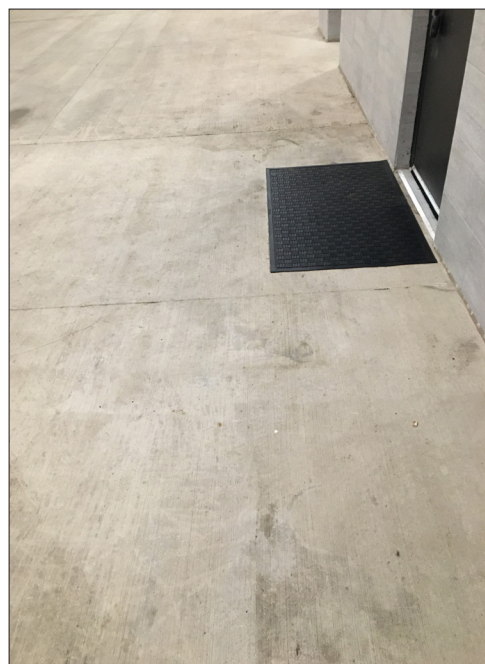
Restaurant walkway after MCI®-2062
